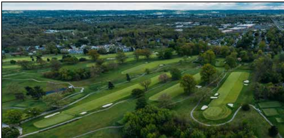
Jeffersonville aerial view
